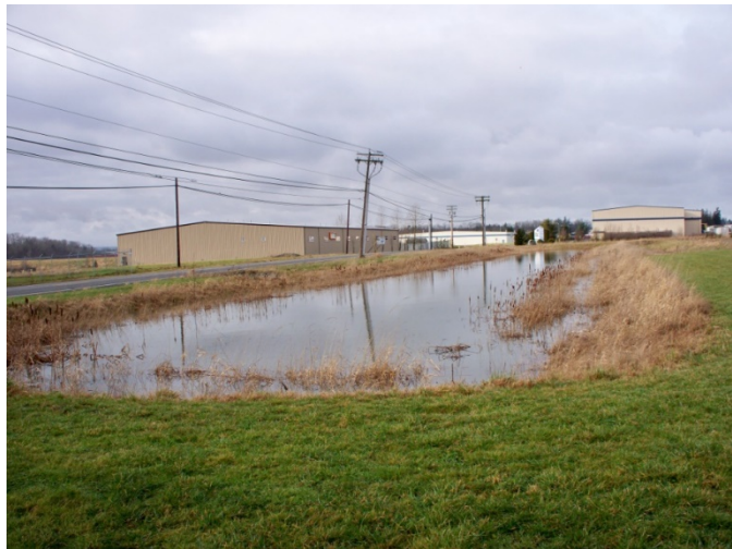
Figure 5: Stormwater Detention Pond
