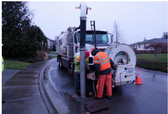
Figure 7: Public Works Crew Using a Vactor Truck
